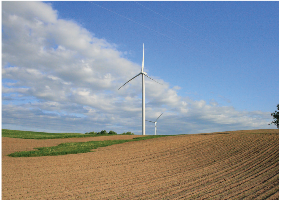
Portland/Slag Cement Construction—Wind Turbine Base
